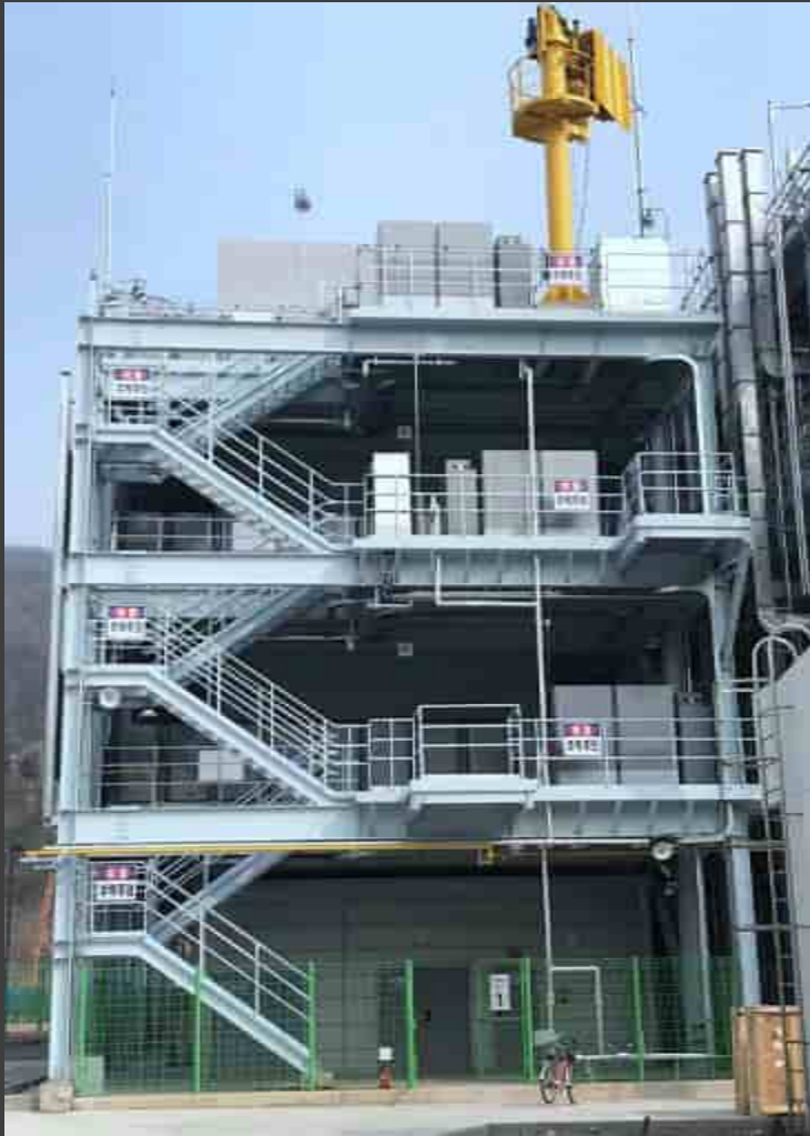
Bundang, South Korea Power Tower Installation
